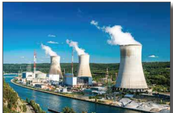
Cooling water control for power plants
